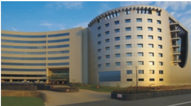
Vascon Weikfield IT Citi Info Park, Off. Nagar Road, Pune
