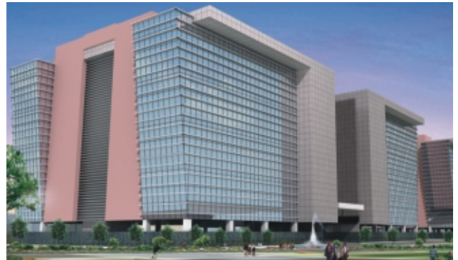
V-Tech - IT / Commercial Park Off Mumbai Naka, Indiranagar, Nashik
